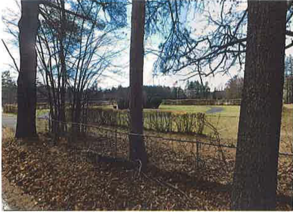
Parcel #: 22 chain link fence Station: 525+50 Rt.
