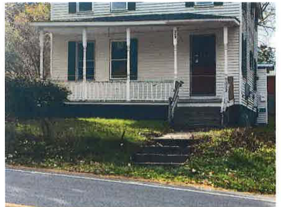
Parcel #: 17 concrete steps Station: 542+35 Rt.
