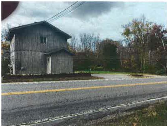
Parcel #: 21 stone and mortar wall and planter Station: 536+90 Rt. & 536+40 Rt.
