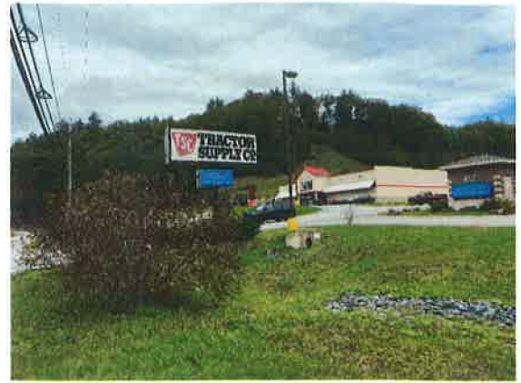
Parcel #: 5C advertising sign and light post Station: 516+60 Lt.
