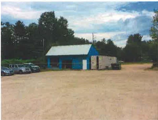
Work shed is the only structure on the parcel.
